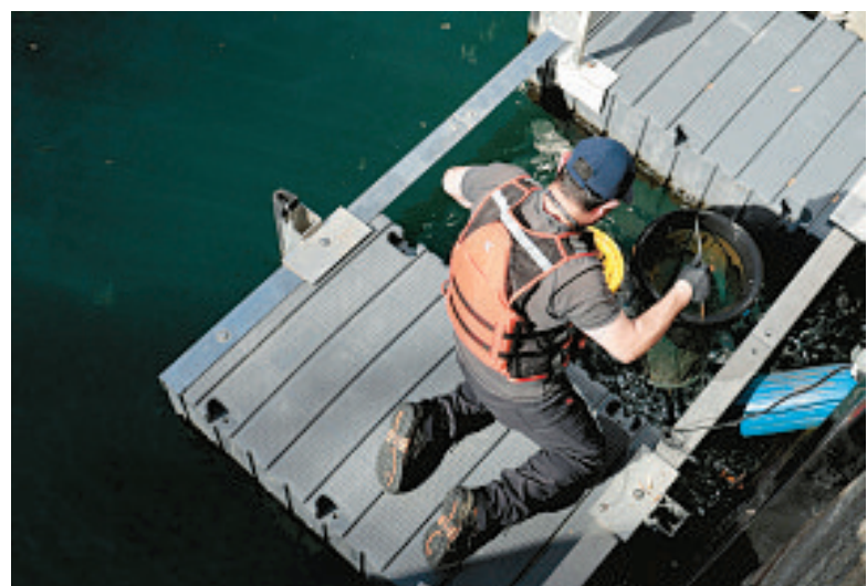
Wendella engineer Miguel Chavez works with the Trash Trap on Wednesday in the Chicago River near Michigan Avenue. The floating trash-collection trap is the first technology of its kind used in the Chicago River to remove litter and learn where it's coming from. ANTONIO PEREZ/CHICAGO TRIBUNE
