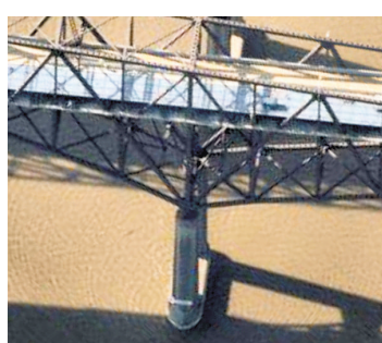
Newburgh-Beacon Bridge, New York
