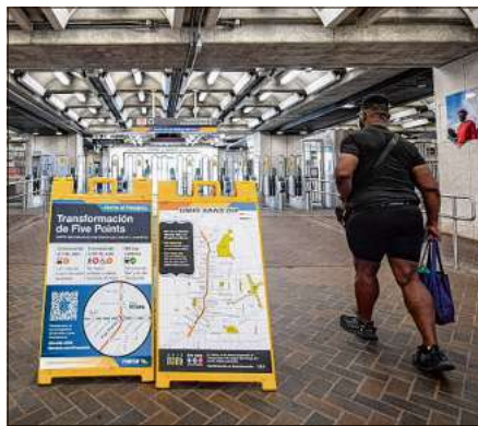
A construction notice is seen in Atlanta's Five Points Station in June. Mayor Andre Dickens denied holding up permits and said the city wants work to start. AJC FILE
